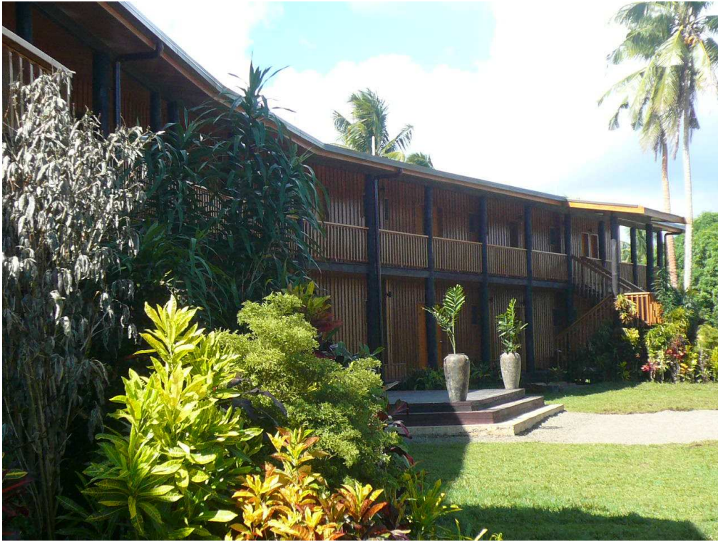
Oneness Lodge accommodation block
